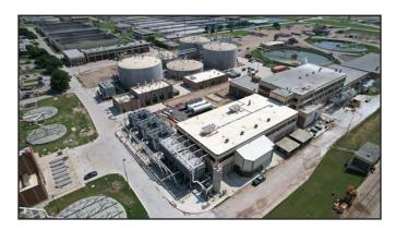
Thermal hydrolysis is a process that heats and pressurizes sludge in order to break down sludge cell walls. This enhances digestion and solids destruction; and consequently, reduces the amount of solids to be moved offsite, thus reducing transportation costs. Biogas production is also enhanced. When used in combination with downstream mesophilic digestion, the process generates Class A biosolids.
